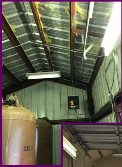
Replaced insulation at Line 1 Impoundment
