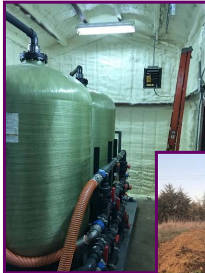
New foam insulation and treatment system at Line 1 Impoundment
