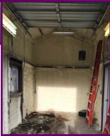
Replaced insulation at Line 1 Impoundment
