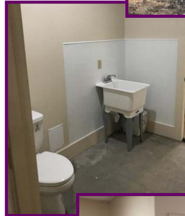
New restroom at IDA
