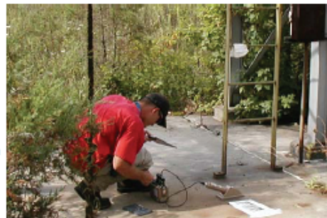
SAIC (FUSRAP subcontractor) performing radiological survey at the Deactivation Furnace.
