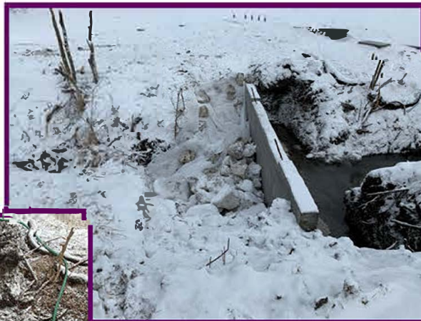
Winter construction included the weir installation
